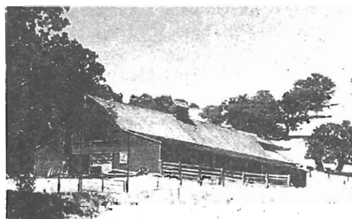
The Schultz Barn
